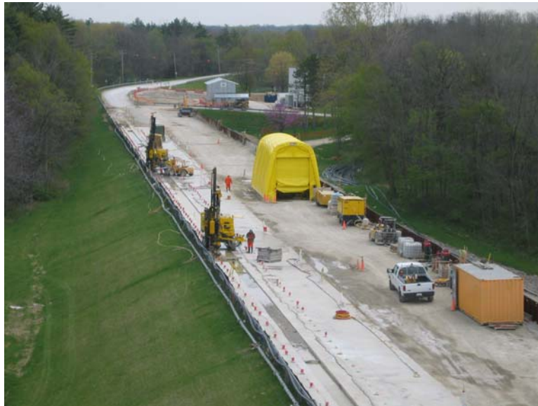
Figure 10. Pregrouting for the Mississinewa Dam, IN Cut-Off Wall.
